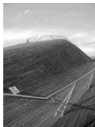
Figure 43 : Terminal de Yokohama – FOA architectes.
